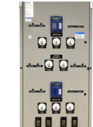
Protective relaying / switchgear door upgrades
