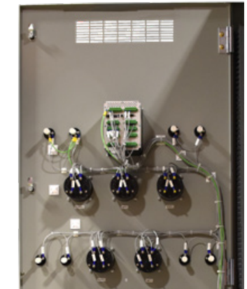
Protective relaying / switchgear door upgrades
